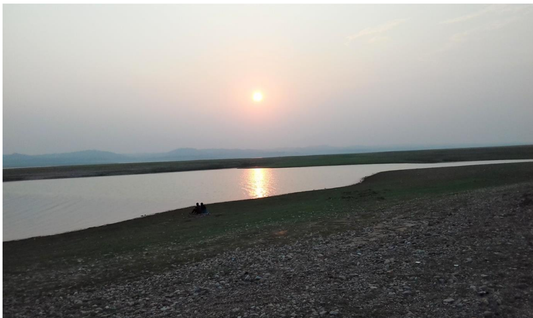
Fig. 2: A view of the Pong dam
