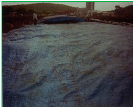
Fig 3 : Use of HDPE sheets (250G.S.M) over the AOSB before the onset of rains during rainy season
