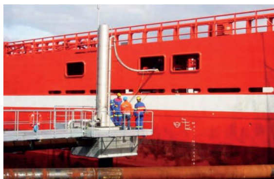
Figure 6. Refueling through the pipeline from the intermediate terminal storage tank to the ship (Eidesvik Norway refueling station)
