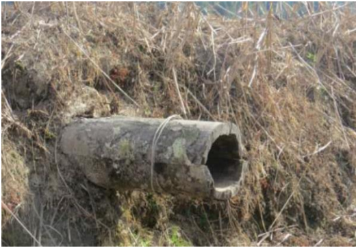
Figure 5. Water outlet made up of bamboo (Uiicho)
