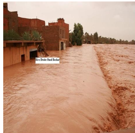
Figure 2. The flood of October 2008 (homes flooded)
